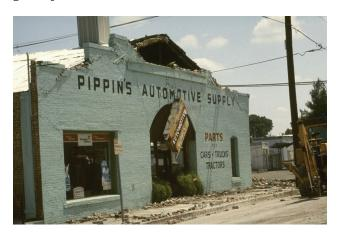
■ Figure 16. URM building with end-wall failure, 1983 Coalinga, California earthquake. Robert Reitherman
