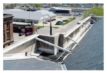
■ Figure 29. Retrofit bracing of an unre-inforced masonry parapet.
