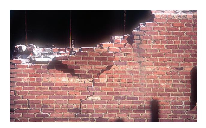
■ Figure 6. Damaged URM wall in a red-tagged building, fated to be torn down or to undergo a multi-year closure for repairs and upgrading.
