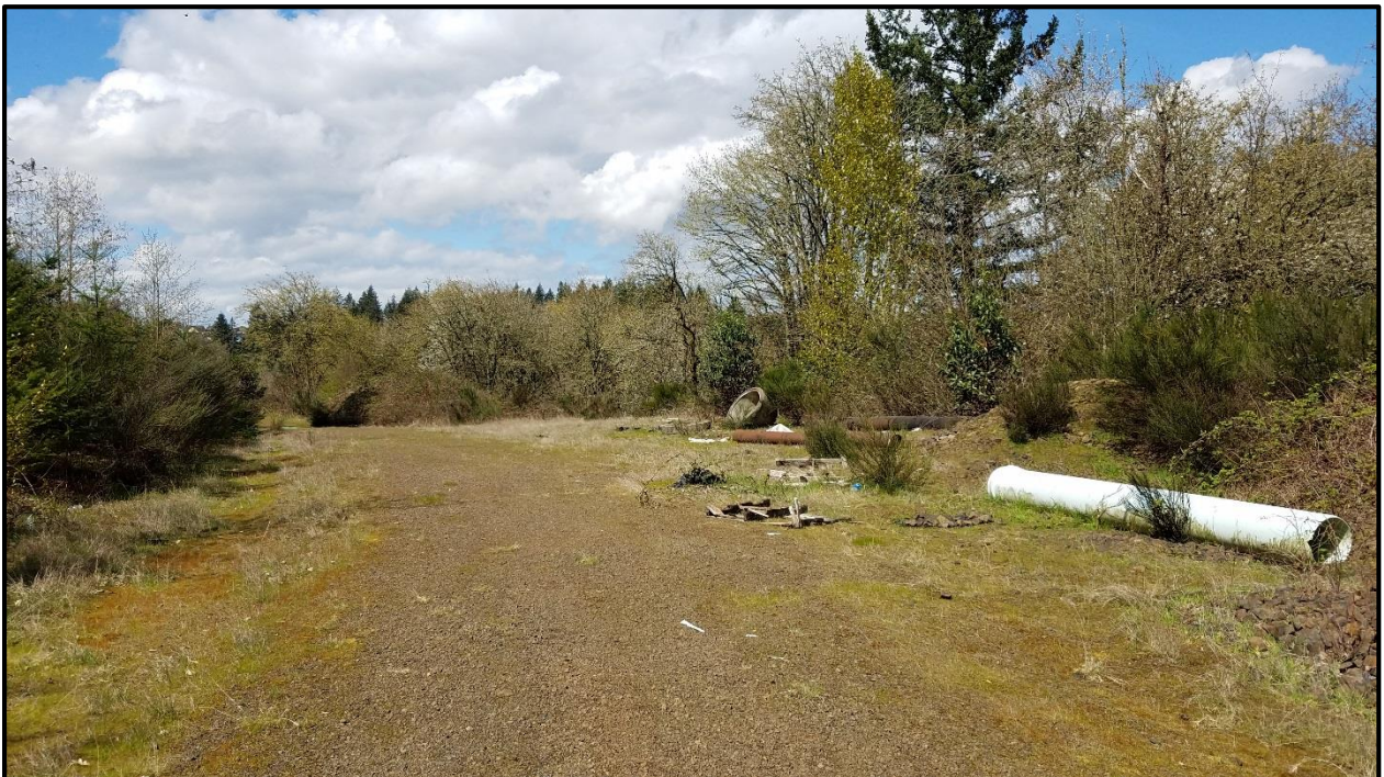
Beyond the barricades, looking north, showing initial grading of Lone Oak Road. [Unused water pipe, sewer pipes, and manhole are on the right edge of the road.]
