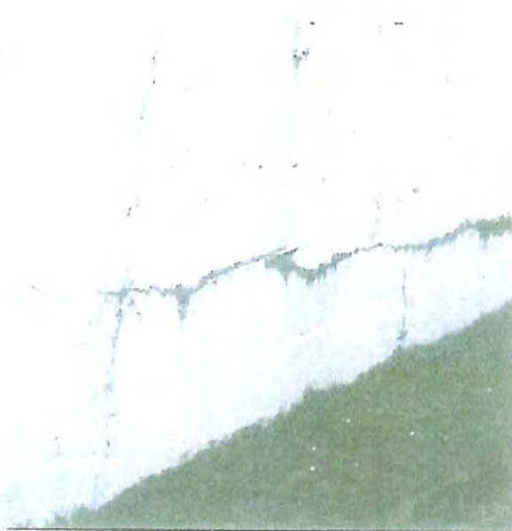
5. Crack in Ramp Wall
