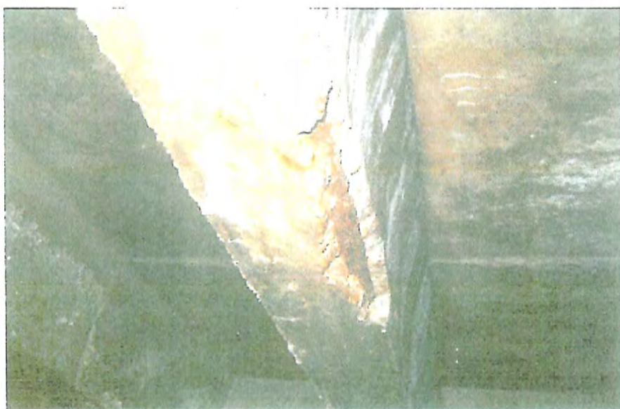
2. Rusting Rebar in Bottom of Concrete Joist
