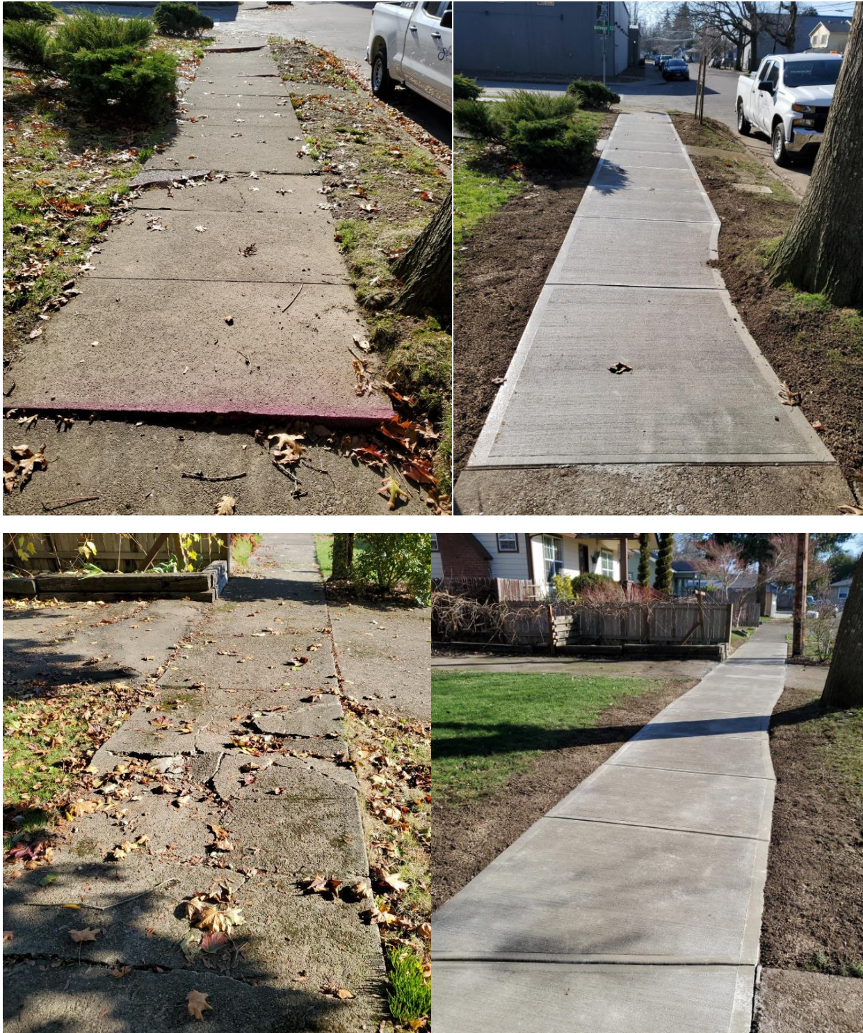
490 21st St SE- 845 Sq ft of sidewalk replaced
