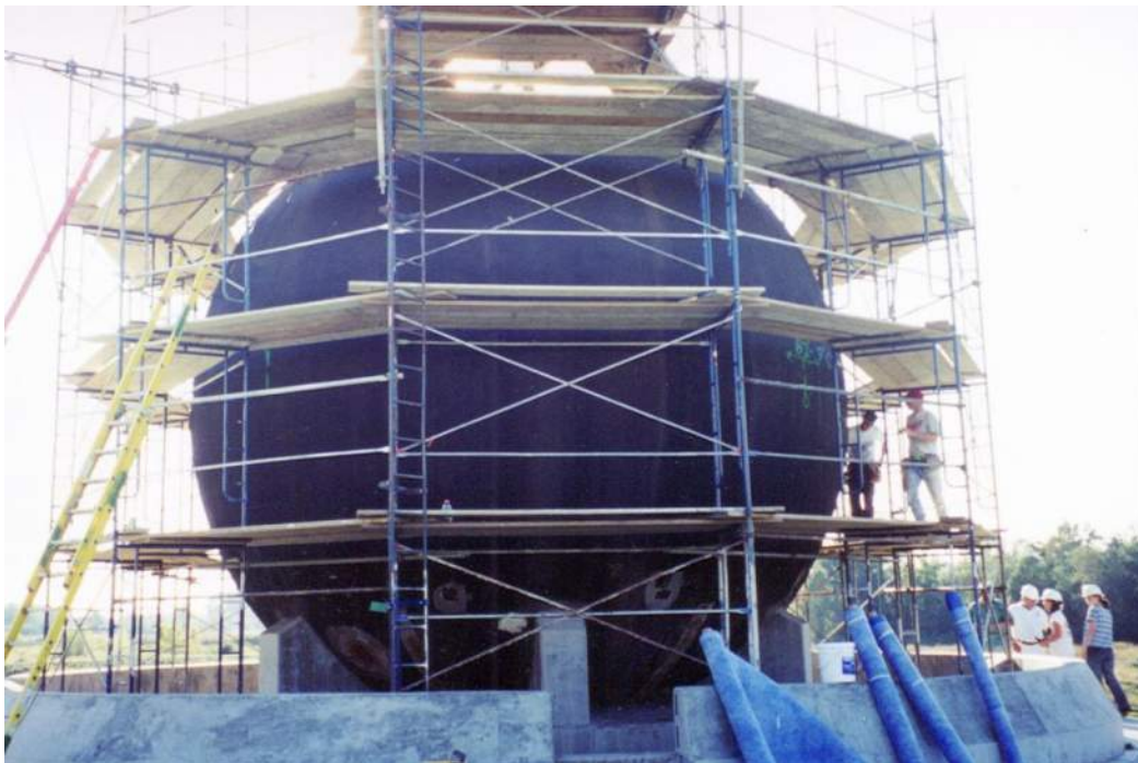
Acid Ball – with scaffolding for installation of tiles- c 2003
