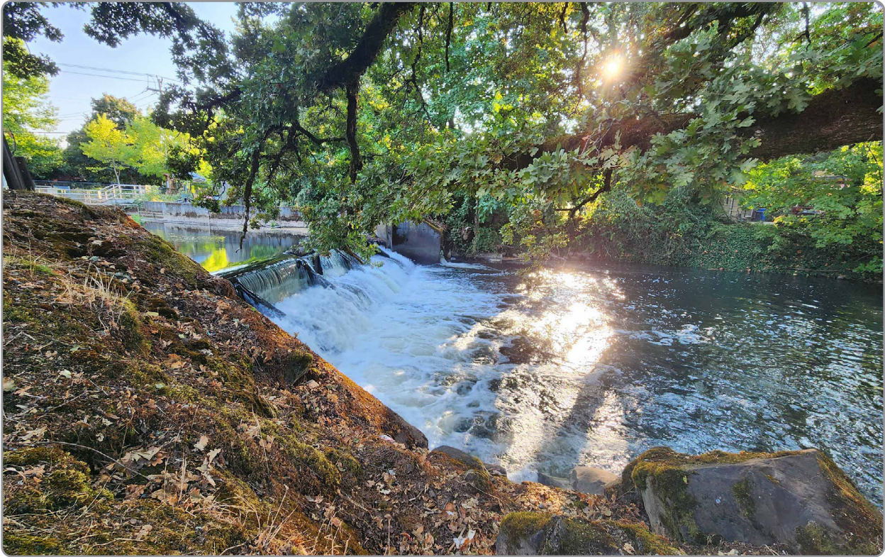
Figure 22: Waller Dam at Shelton Ditch (North Santiam Watershed Council, 2025)
