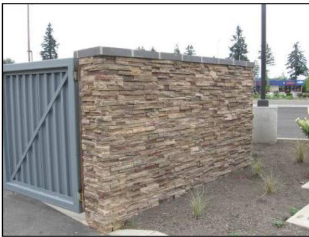
FIGURE 534-8 GROUND-LEVEL MECHANICAL EQUIPMENT
