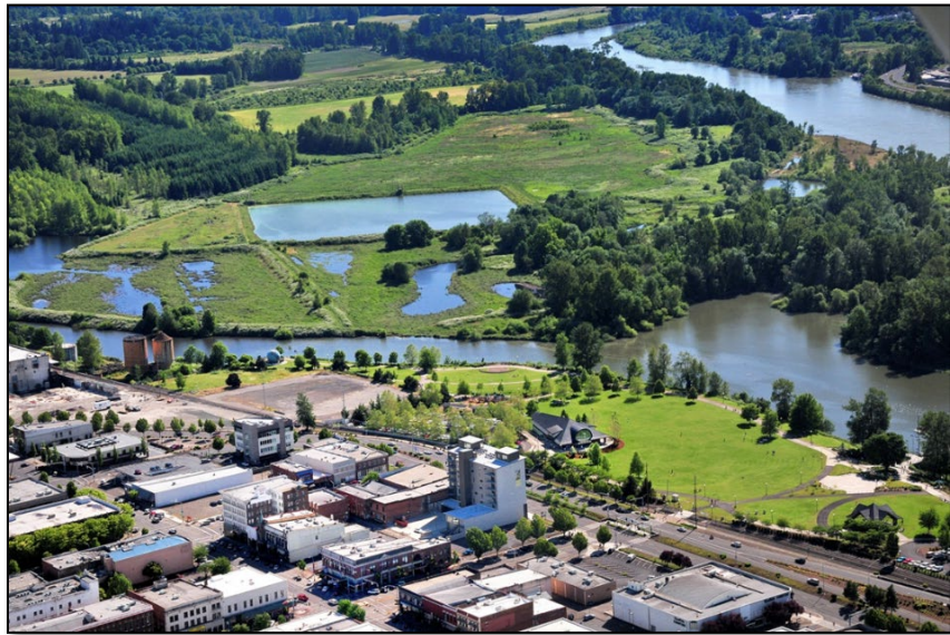
Figure 5. Aerial view of MICA from around the time of the City's acquisition (c. 2013, prior to construction of the pedestrian bridge).
