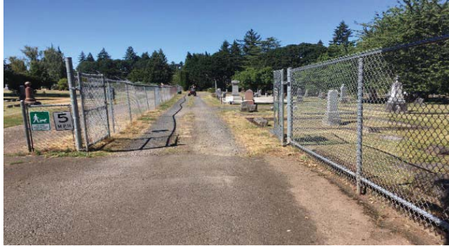
Current South entrance gate
