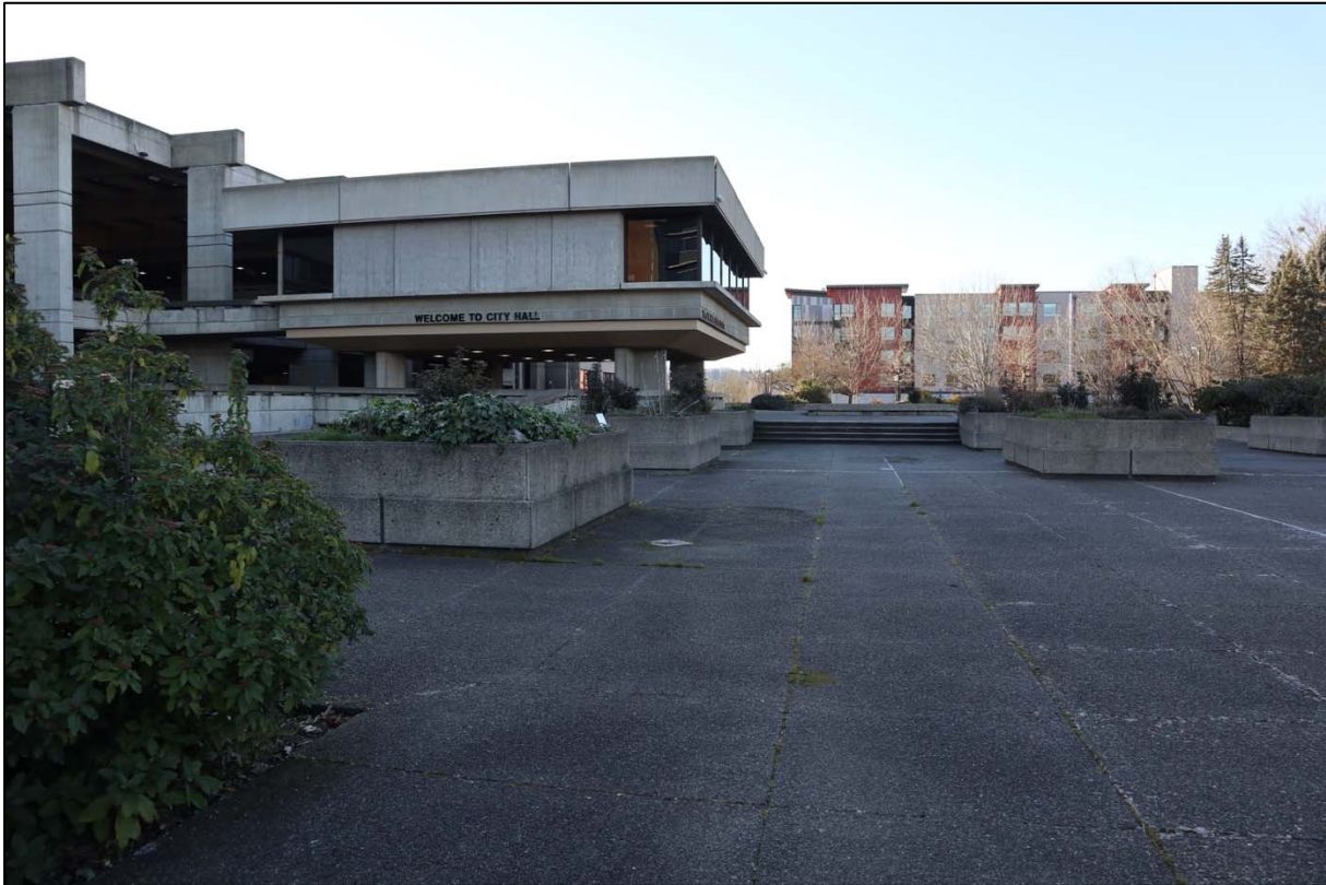
Photo 13 of 40. City Hall Council Chambers and landscaping, looking west.
