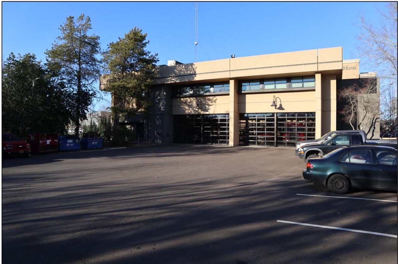
Photo 4 of 40. Central Fire Station #1 south elevation, looking northwest.
