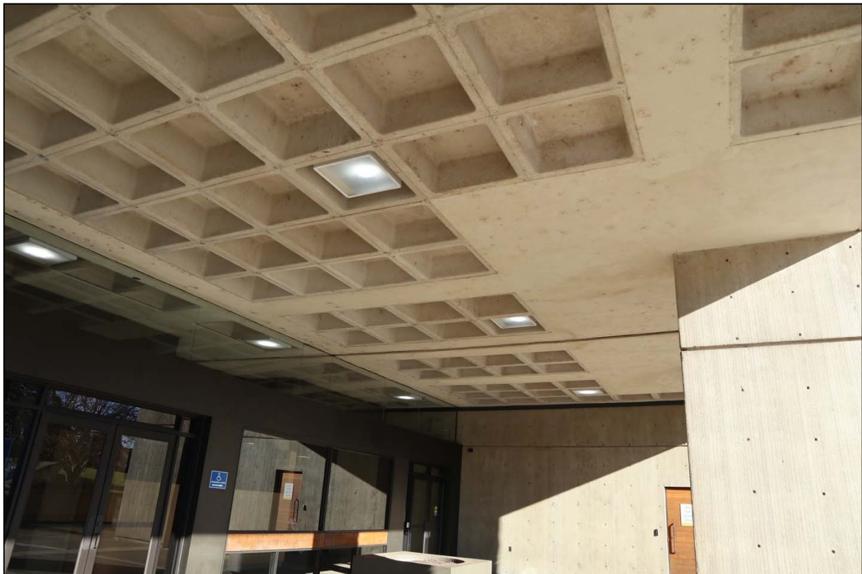
Photo 20 of 40. City Hall waffle slab construction in the front entry, looking east.
