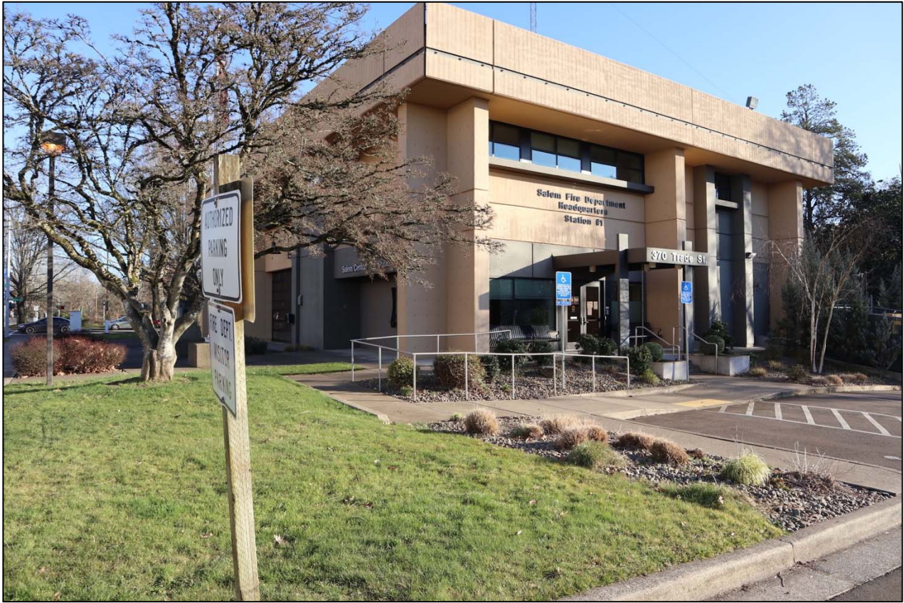
Photo 1 of 40. Central Fire Station #1 west elevation, looking southeast.
