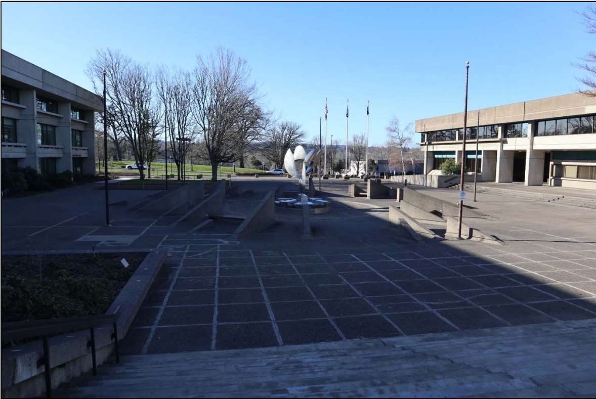
Photo 27 of 40. Plaza Fountain, looking west.
