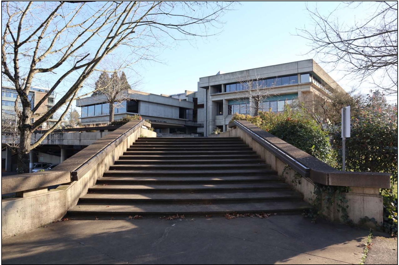
Photo 36 of 40. Staircases leading to City Hall, looking southeast.
