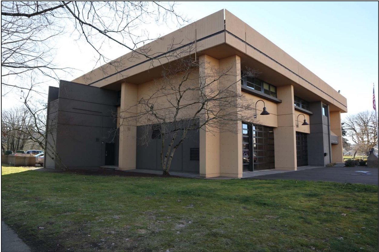
Photo 3 of 40. Central Fire Station #1 north and east elevations, looking southwest.
