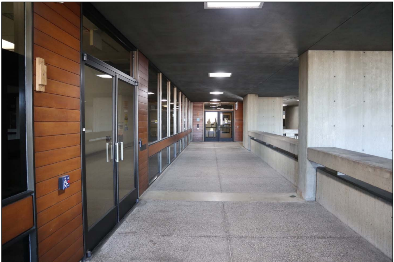
Photo 22 of 40. City Hall example of offices, looking northwest.
