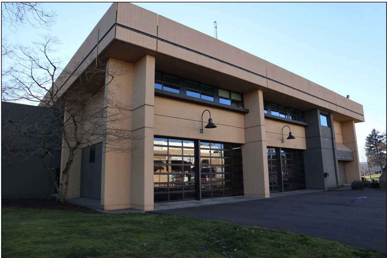
Photo 2 of 40. Central Fire Station #1 north elevation, looking southwest.
