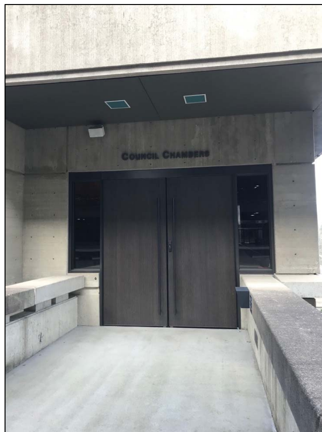
Photo 37 of 40. City Council Chamber doors, looking north.
