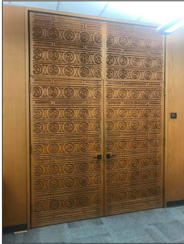
Photo 38 of 40. City Hall Mayor's Office Doors, looking south.
