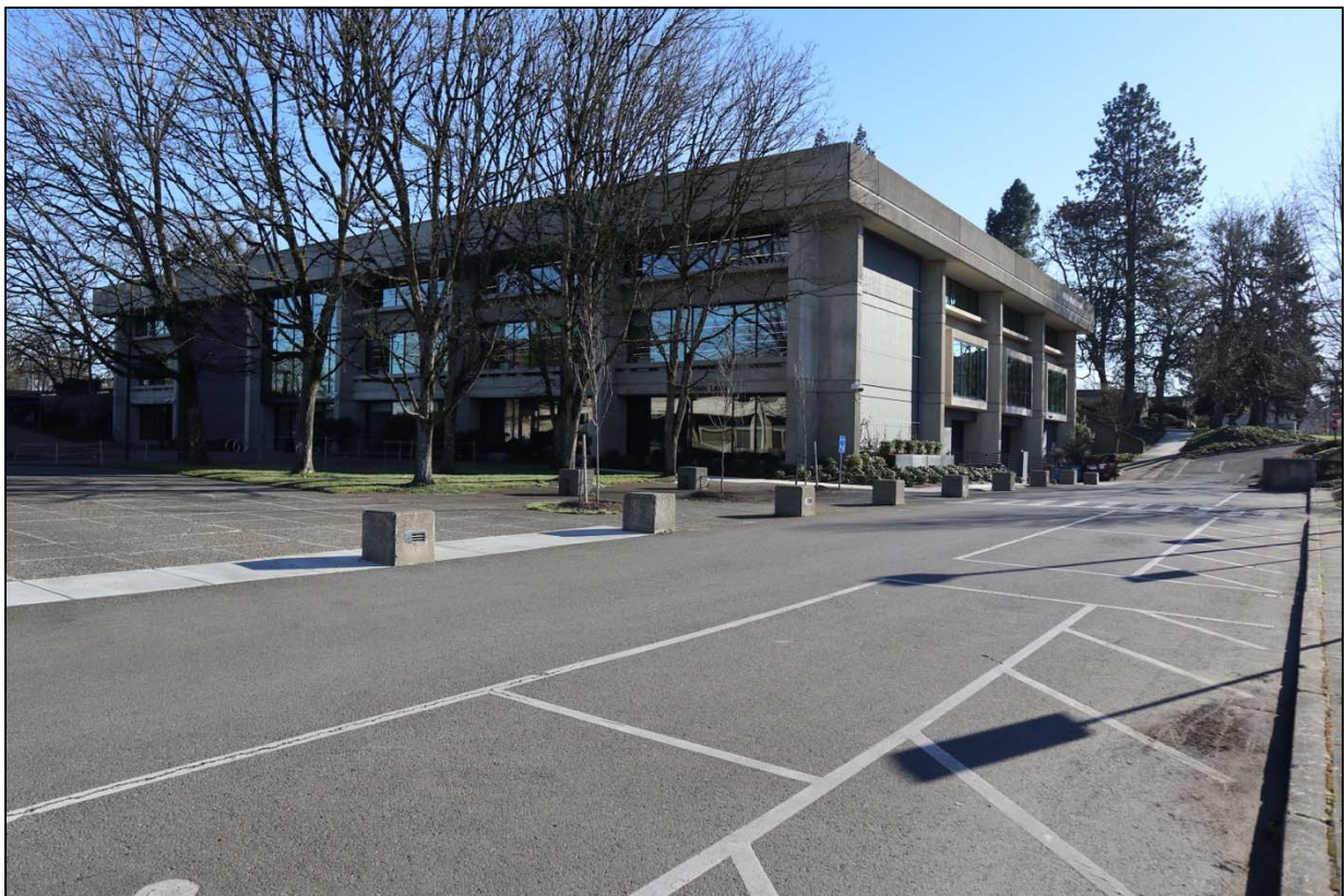
Photo 30 of 40. Public Library north and west elevations, looking southeast.
