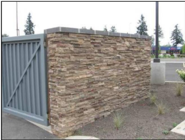
FIGURE 534-9 ROOFTOP MECHANICAL EQUIPMENT
