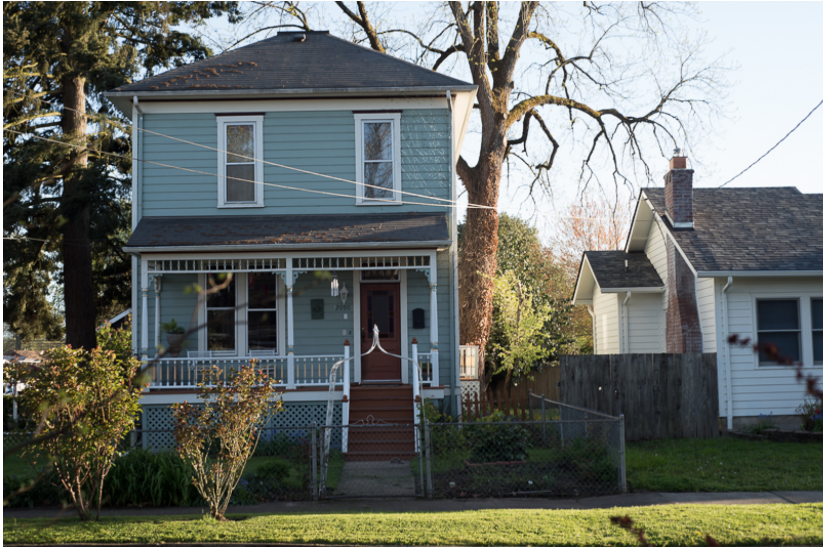
Photograph 8: Court Street NE at 21st Street
