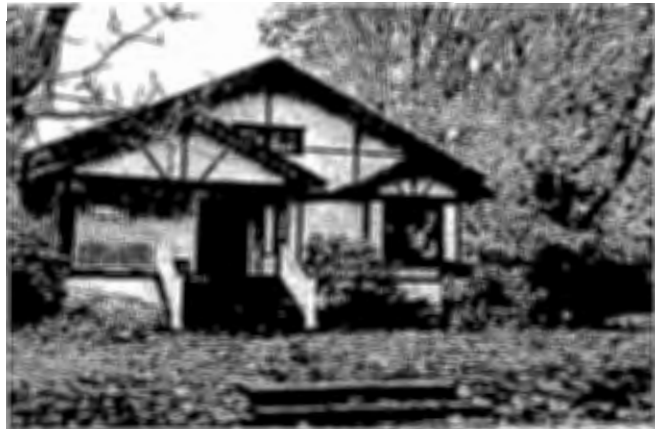
1566 Court Street (Fall 2017)
