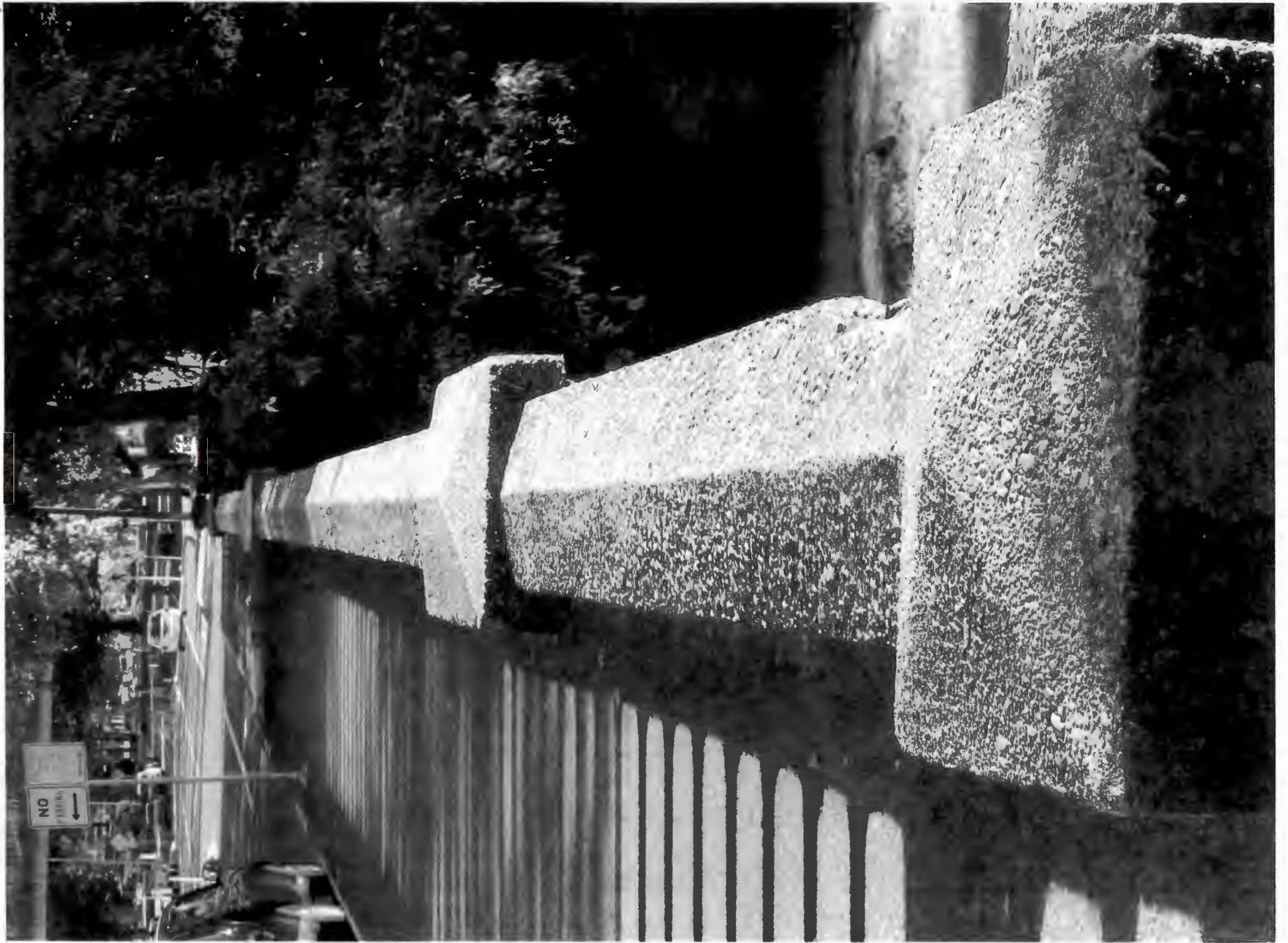
Balustrade without shading from vegetation
