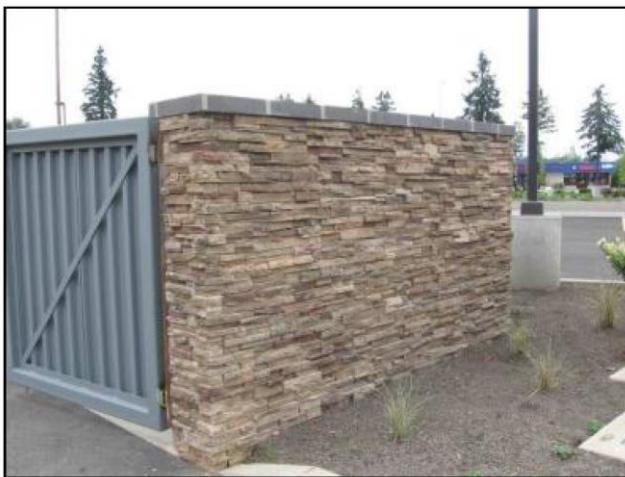
FIGURE 534-8 GROUND-LEVEL MECHANICAL EQUIPMENT
