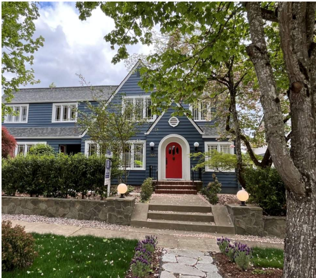
460 Bush St SE after restoration
