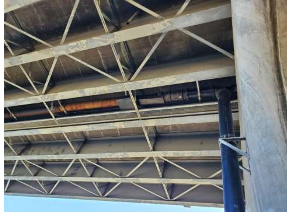
Infrastructure Upgrades: City waterline
