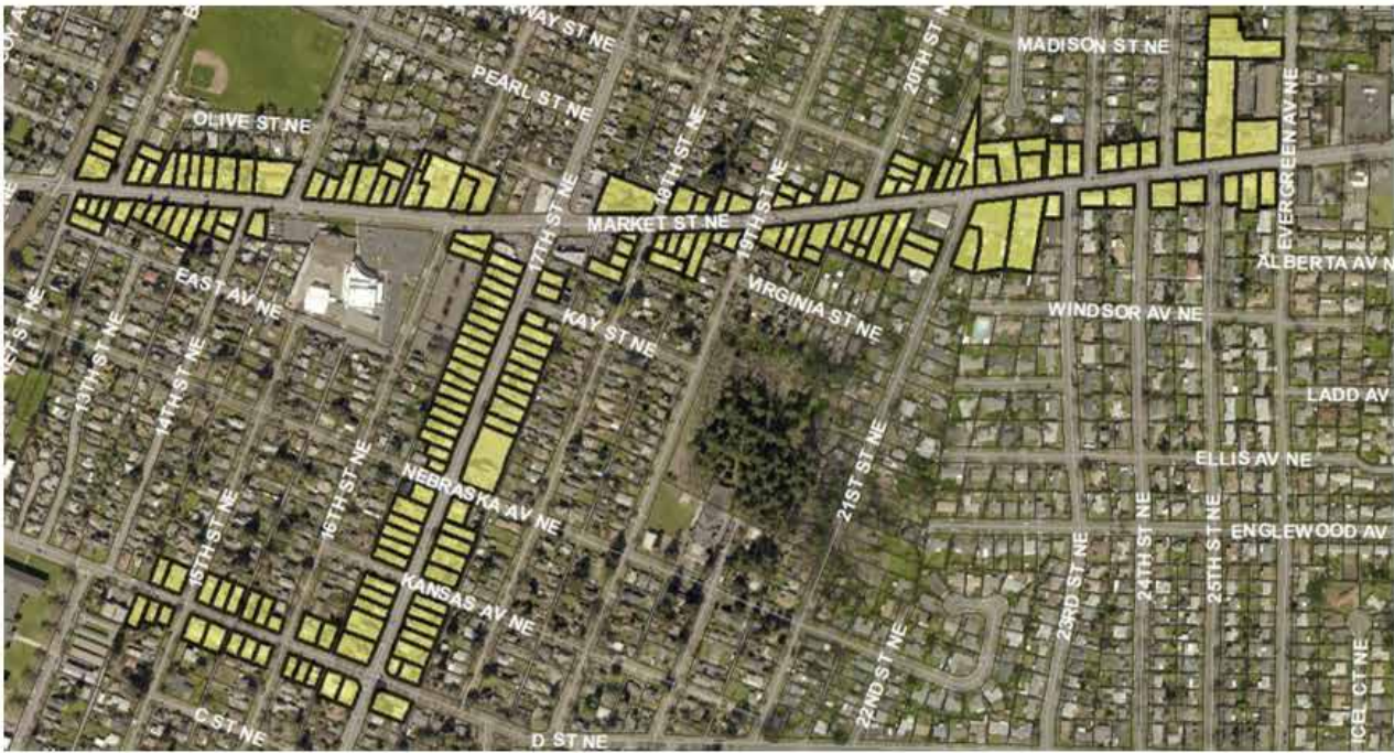
Market Street NE between Garnet Street NE and Evergreen Avenue NE; 17 th Street NE from D Street NE to Market Street NE
