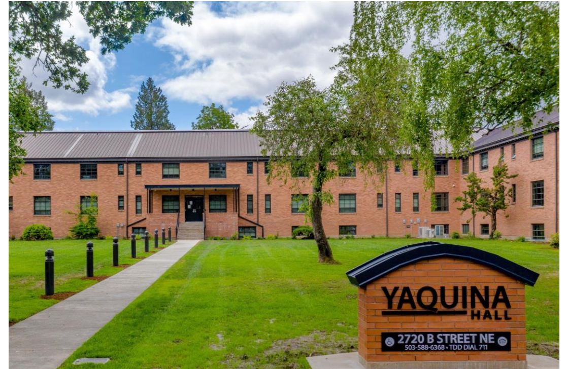
Yaquina Hall Rehab
