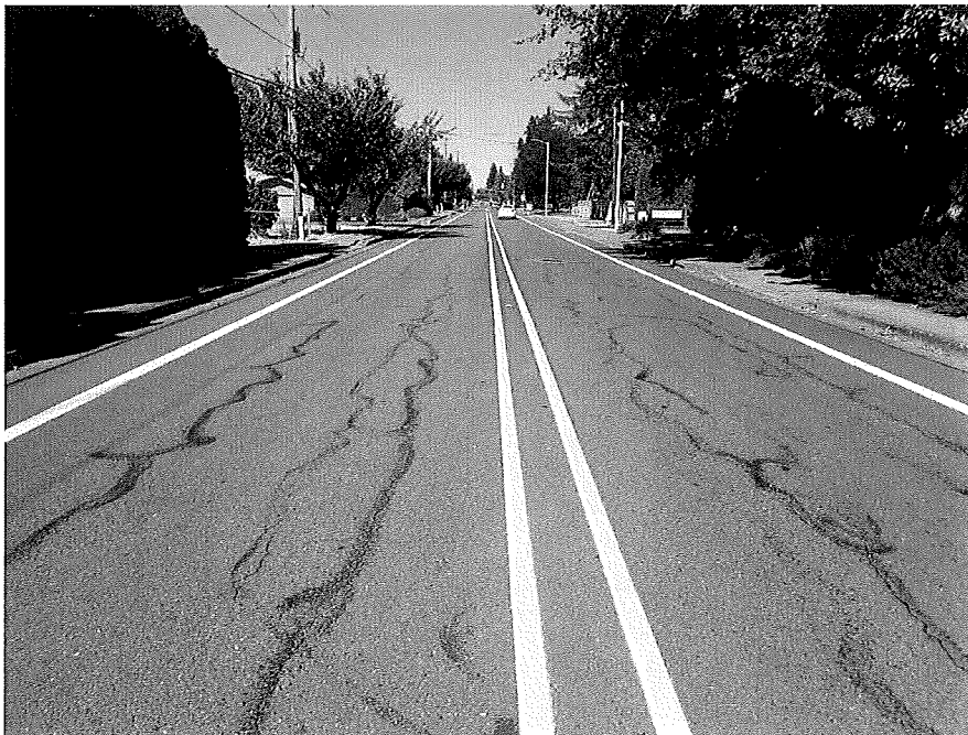
6. Looking north from 100 feet north of Thrush Drive.
