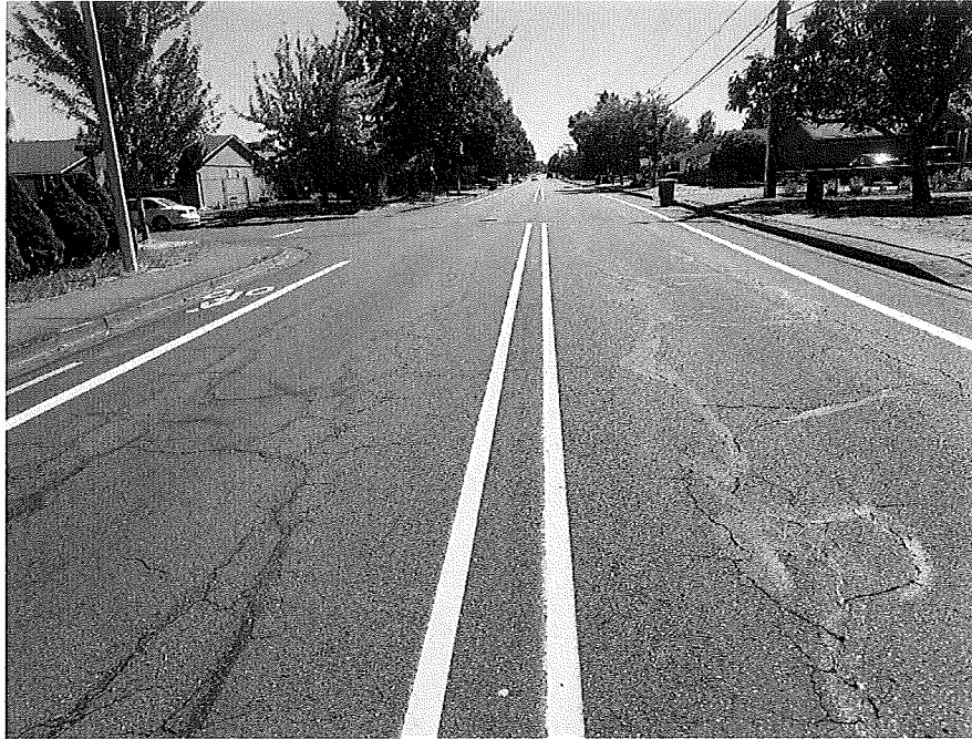
5. Looking south from 100 feet north of Thrush Drive.
