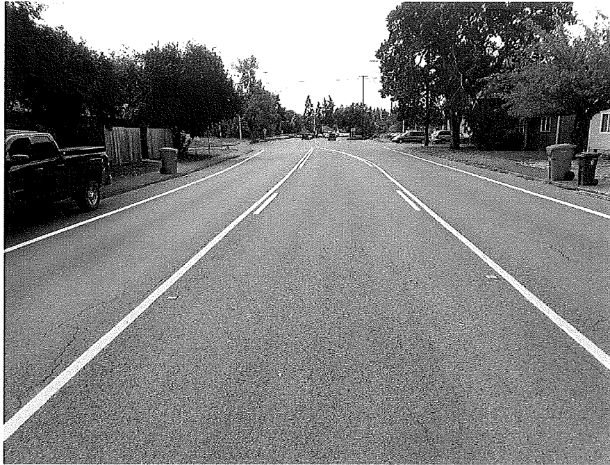
1. Looking south from 150 feet north of Oak Street.
