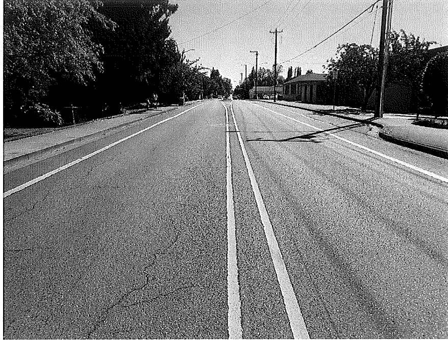
9. Looking south from 200 feet south of Country Lane.
