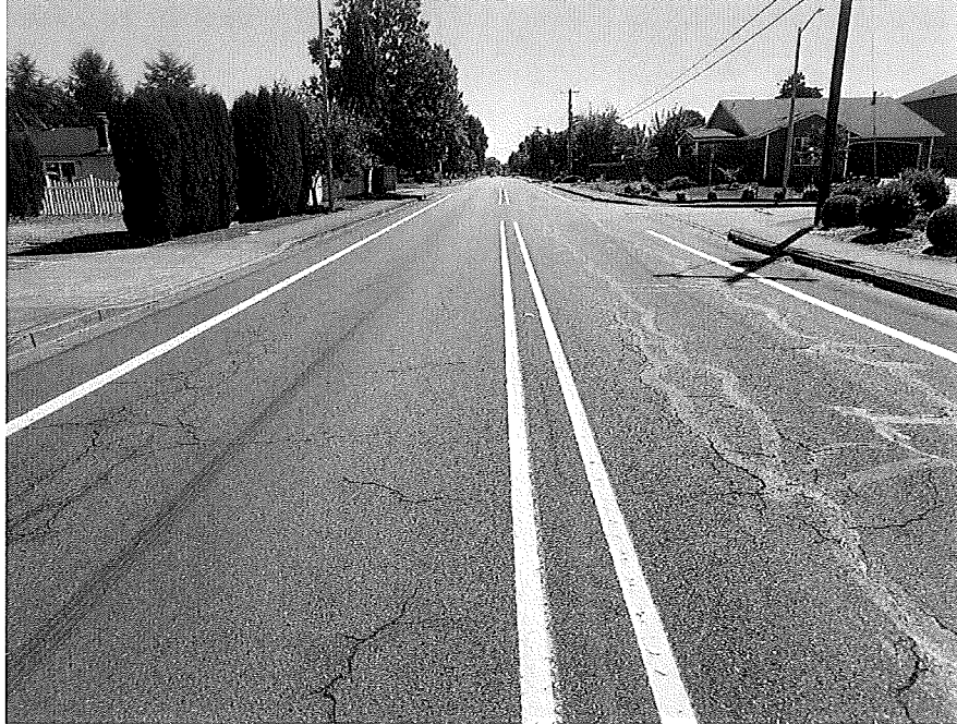
3. Looking south from 100 feet north of Dean Street.
