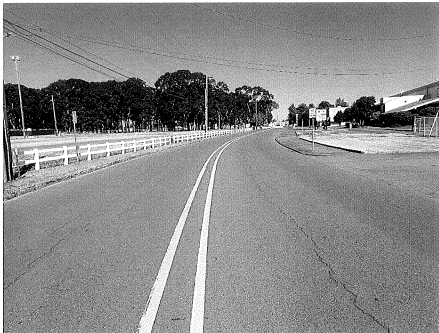
22. Looking north from 150 feet north of Woodrow Street.
