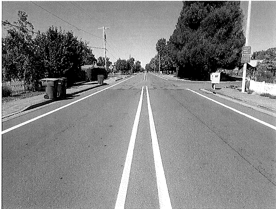
2. Looking north from 100 feet south of Beth Street.
