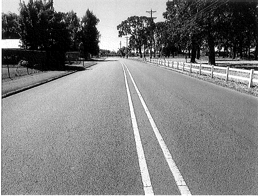
23. Looking south from 350 feet south of Silverton Road.
