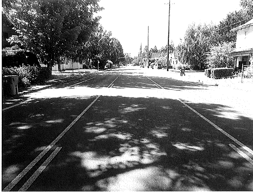
13. Looking south from 150 feet north of Kansas Avenue.
