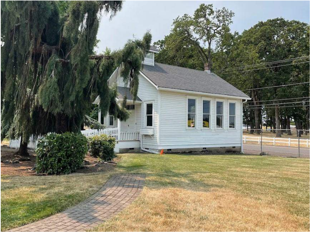
Image 11: Image of Criterion Schoolhouse taken from the northeast. Source: Ryan Prochaska 2023.
