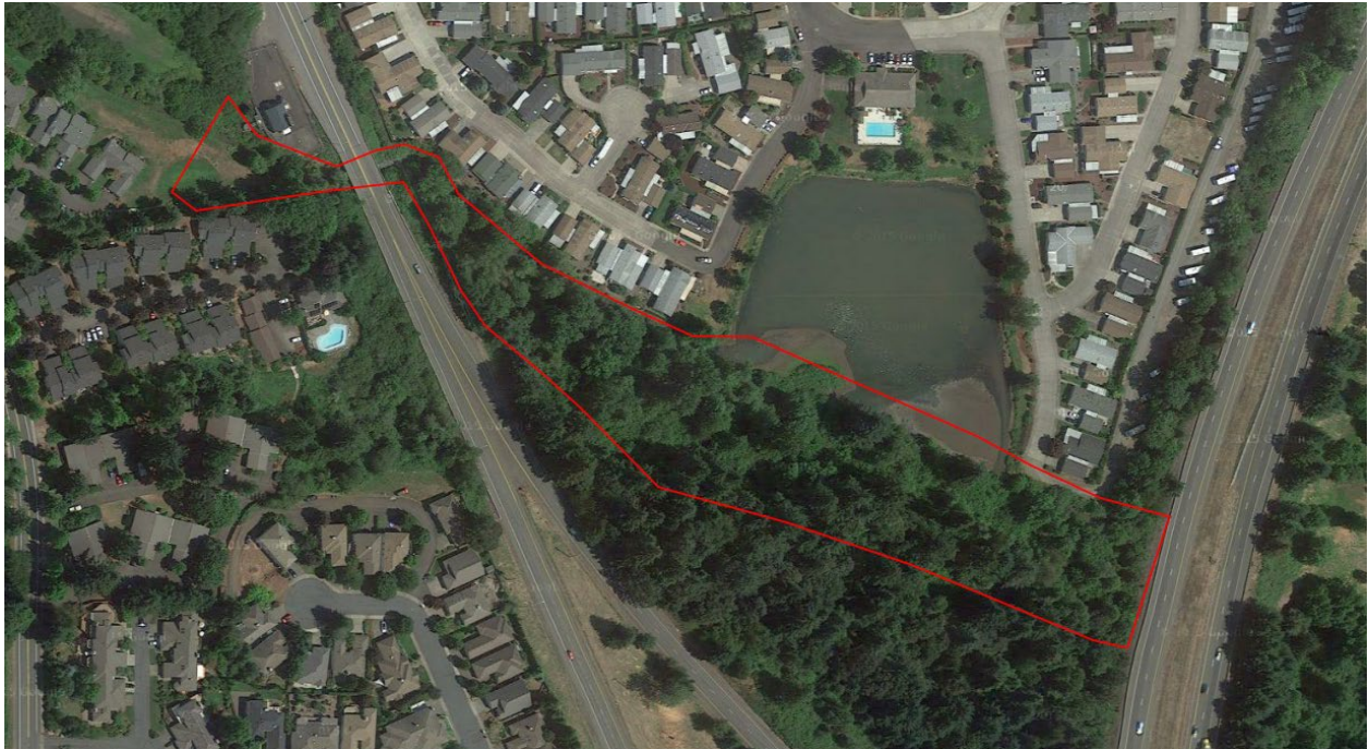
Aerial view of approximate project limits.
