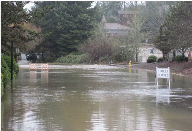
Figure A.7—Flooding at the Madras Street crossing over Waln Creek.
