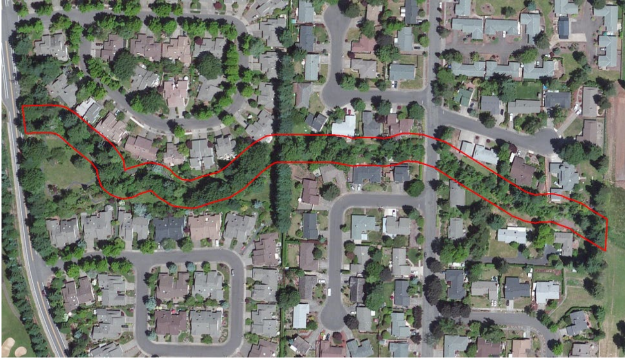
Aerial view of approximate project limits.
