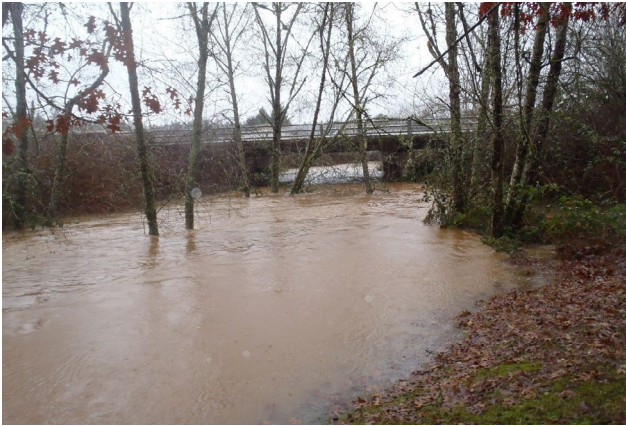
Figure A.1—Across from the BAT3 flow gauge, looking downstream at Commercial Street Bridge.
