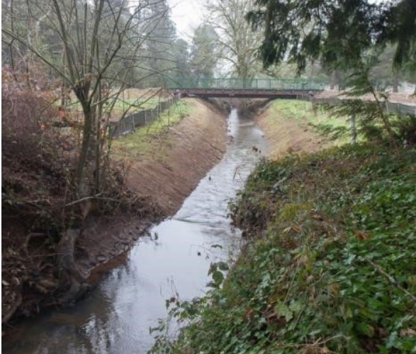
Upstream end of project facing downstream.
