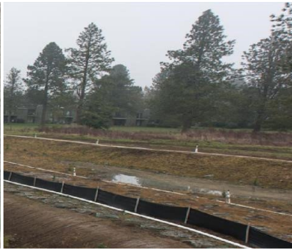
View of floodplain area east of Waln Creek.
