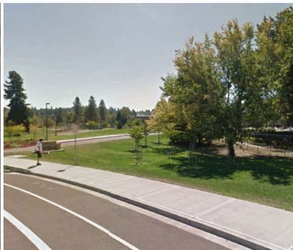
Proposed culvert location at access road.
